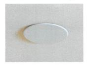
Modern fire sprinklers are inconspicuous and can be mounted flush with walls or ceilings.
